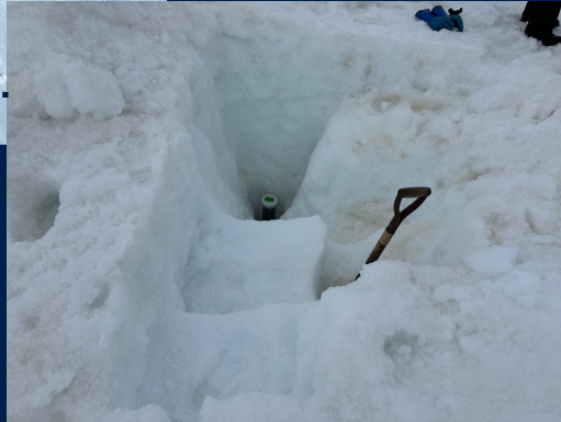
Installation of communication penetrator below the snow surface.
